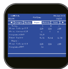
UPS Cabinet Control Panel
